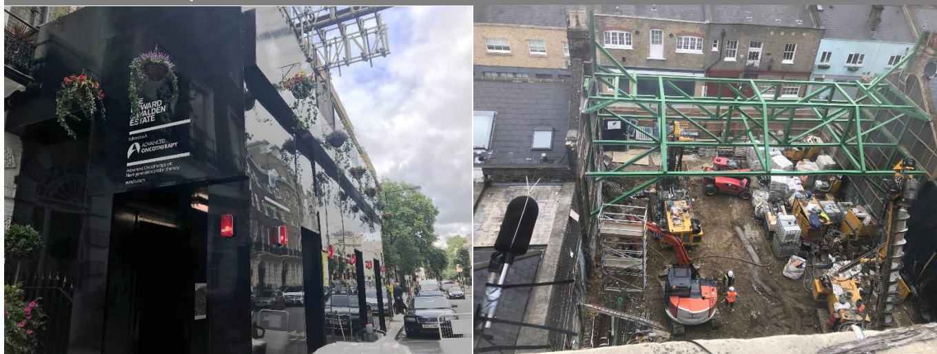
Construction at Harley Street
